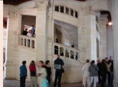
Double helix scale, which allows two people to climb at the same time without crossing at any time.
