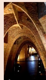
Attic. Parabolic vaults. The roof resembles the ribs of a huge animal
